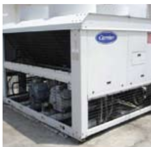
Fig. 2.7 Older standard air-cooled chiller manufactured in Europe with R-22, installed in Montenegro.
