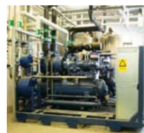
Fig. 2.13 Low charge ammonia chiller with dry expansion, welded plate heat exchangers and a variable speed drive on the compressor.
