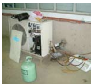
Fig. 2.1 Service of a split system rarely includes recovery in most Article 5 countries. “Release, service and recharge” is common, but should be avoided.
