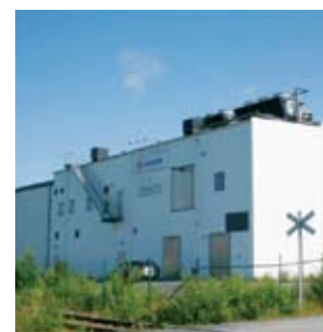
Fig. 2.12 The cold store. The “dry” coolers are on the roof and the low charge ammonia chillers inside.
