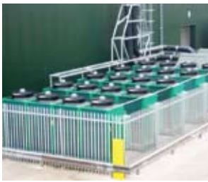
Fig. 2.11 Five air cooled chillers with potassium acetate as brine and hydrocarbon R-1270 as refrigerant.
