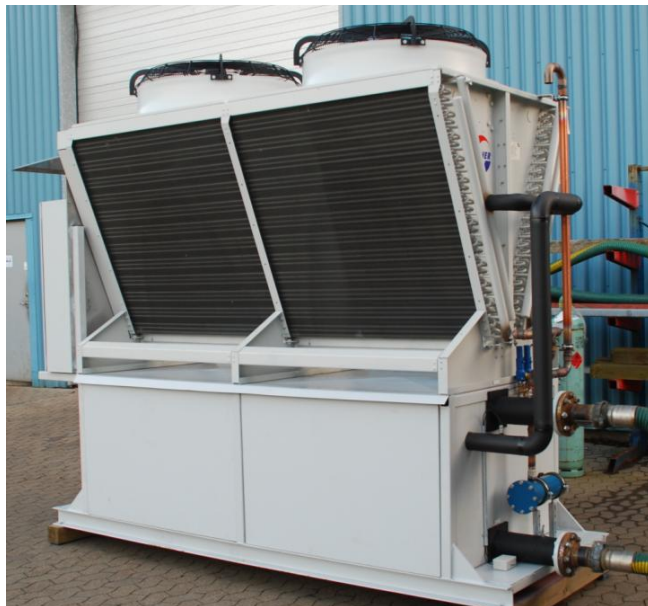
An inverter driven, screw, air-cooled Propane [R290] chiller on test
