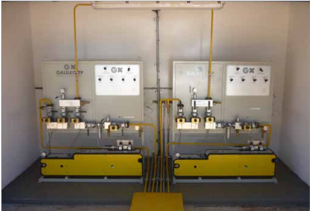
Figure 11: HC feeding system
