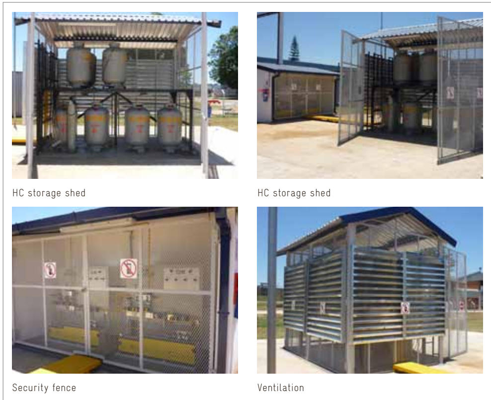
Figure 8: HC storage shed
