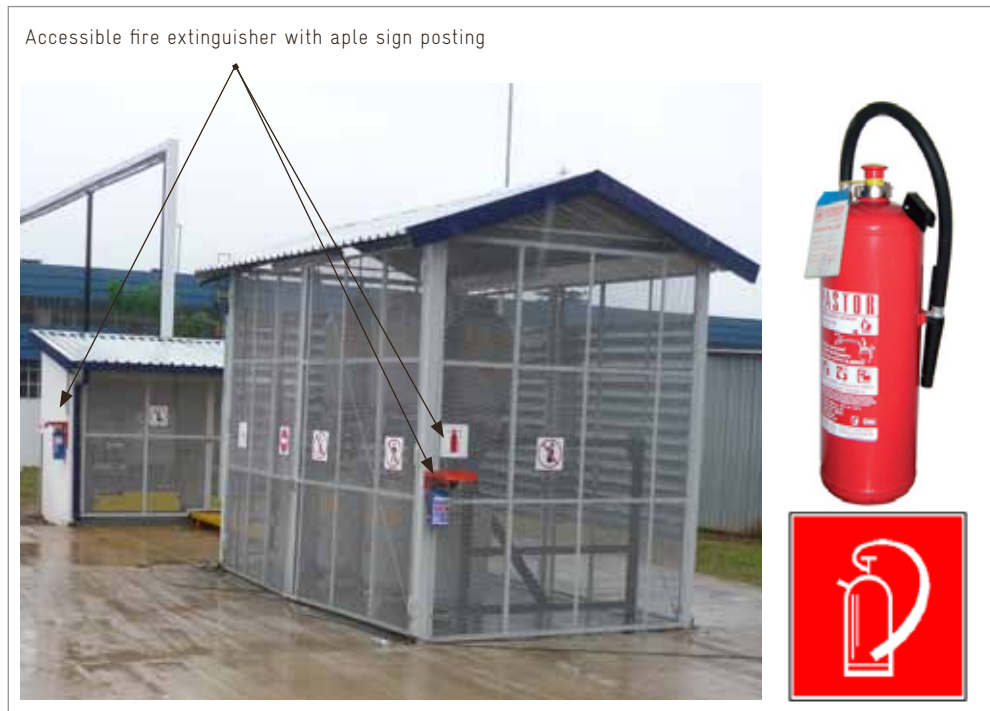
Figure 10: Fire protection for outdoor HC storage
