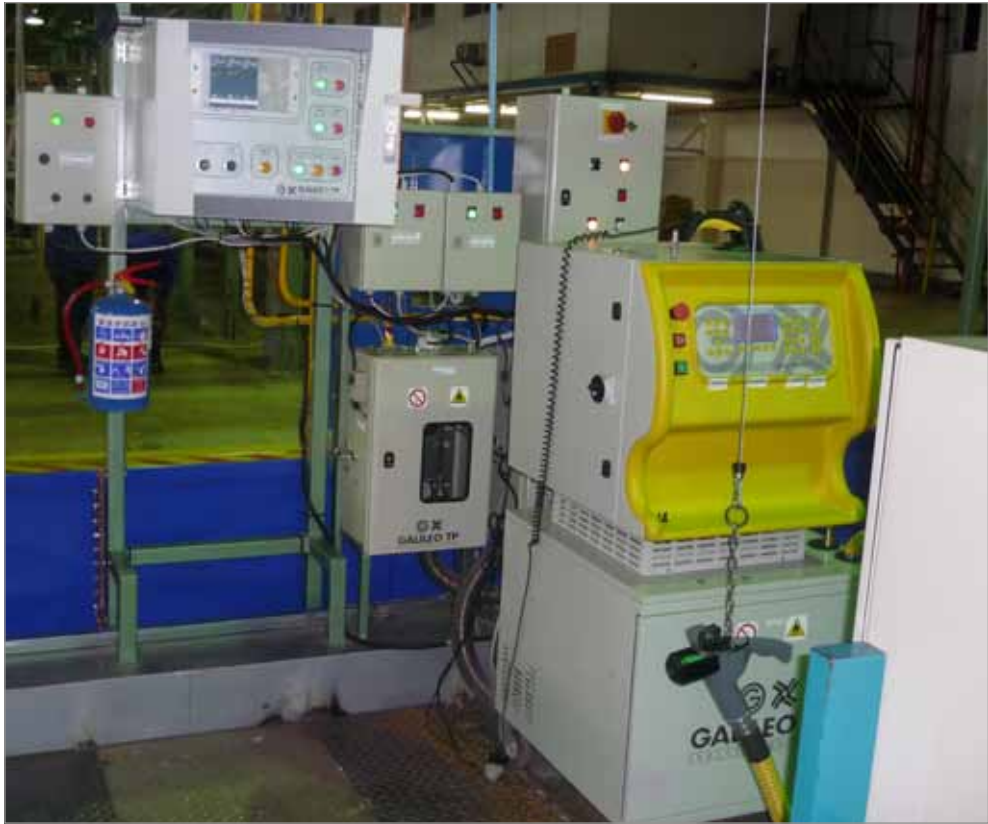
Figure 17: Pumping system in the evacuation area
