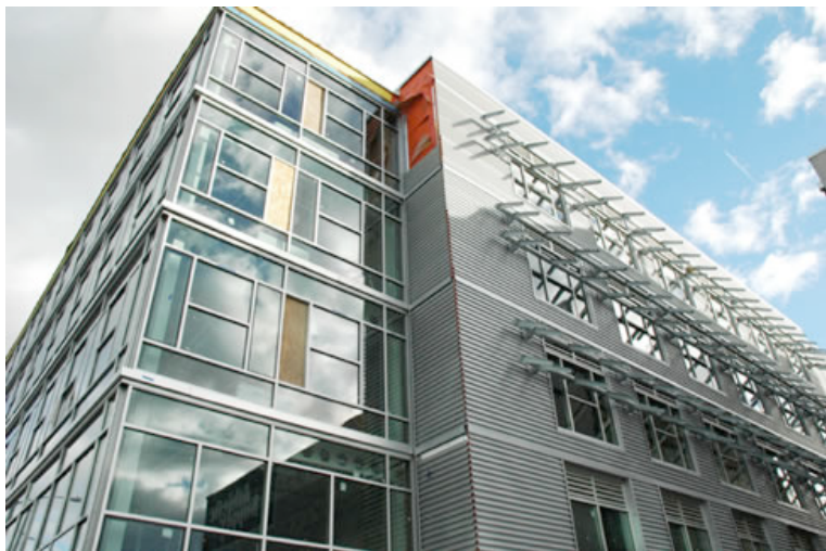
Office building in Seattle, Washington, USA designed by Weber & Thomson requires no air-conditioning. The building has green-tinted glass shades (or sunglasses) that shield windows from heat, while still allowing light into the building. Heat-reflective coating on the windows also reduce temperatures. The 40,000 square foot structure has a central courtyard, which allows cross breezes to enter all parts of the building, and allows more natural light into the building. 66
