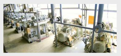
and processing purposes from -41°C up to -5°C. Excellent efficiency and performance results for single stage screw compressors reaching temperatures of -30°C or higher, and two-stage or compound screw compressors generating temperatures of -41°C, were obtained.
