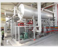
The products are frozen at a temperature of around -40°C in two air-cooled batch freezers. Also a chilling tunnel for cooling the freshly killed chicken uses  $CO_2$  circulated at -10°C and a tunnel temperature about +1°C. A falling film ice water cooler is cooled with  $CO_2$  at -10°C.
